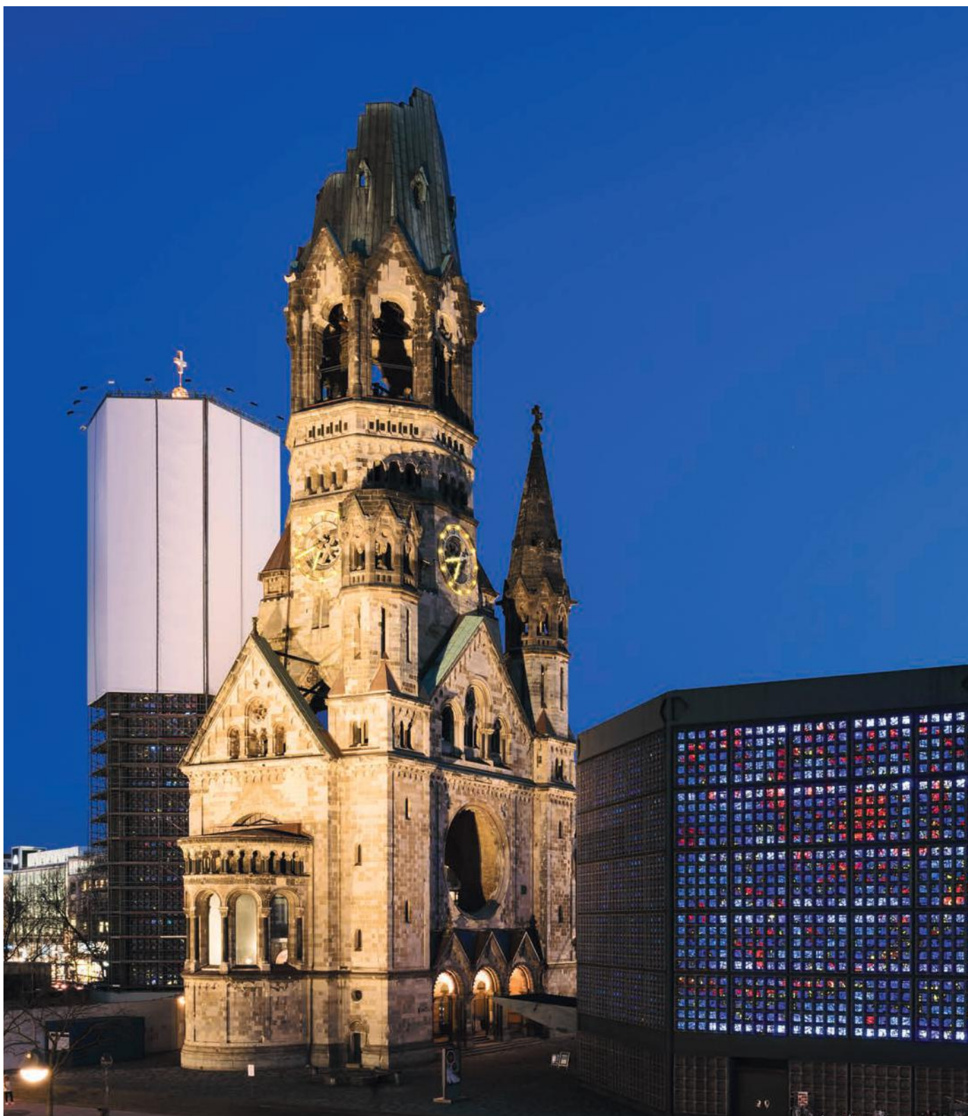
Memorial Church, Berlin, Germany. Luminaire: 49. Light planning: Kardorff Ingenieure Lichtplanung GmbH ©Linus Lintner
