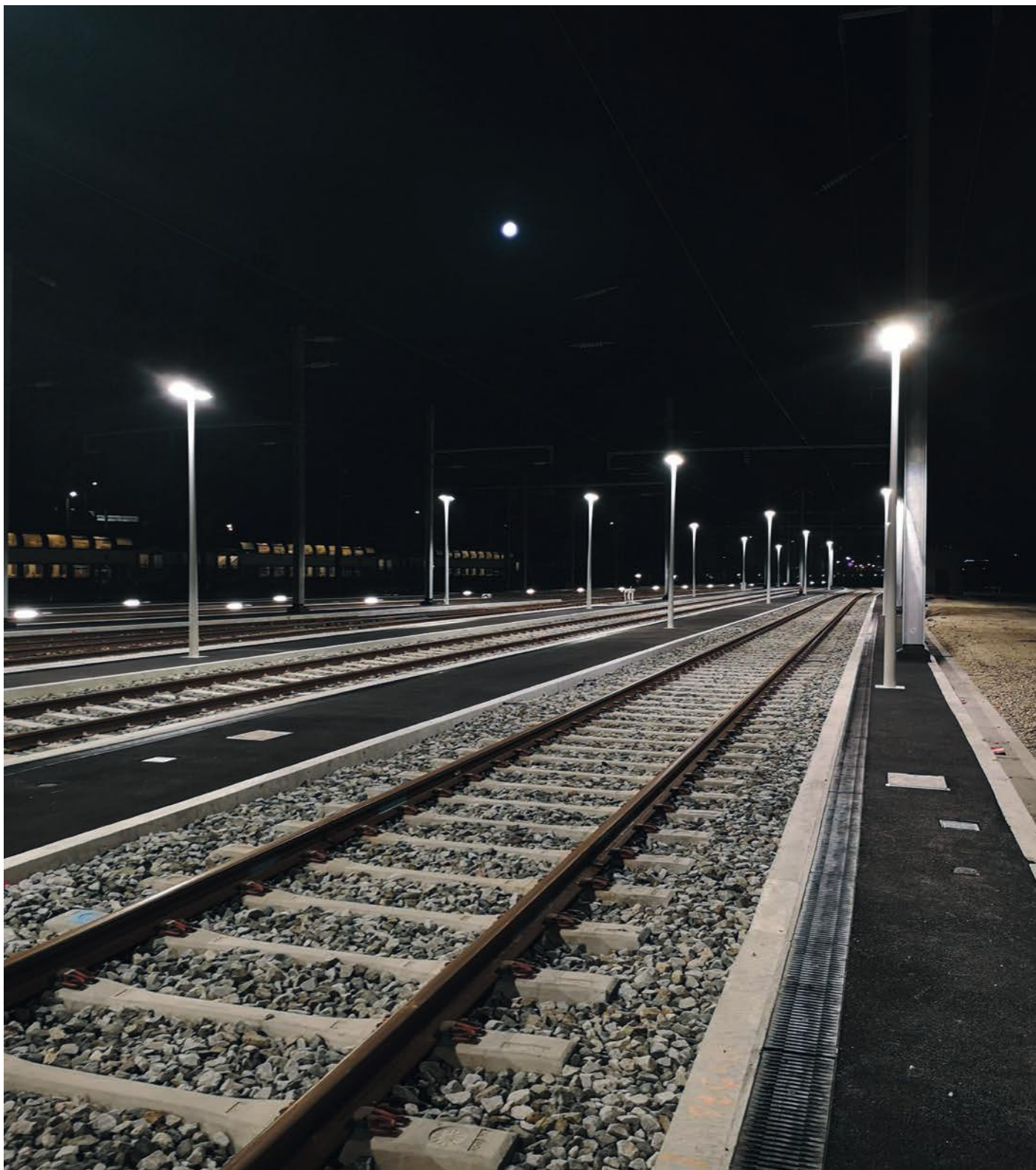
SNCF maintenance system, Dreux, France. Luminaire: 153 ©Frédéric Grazini
