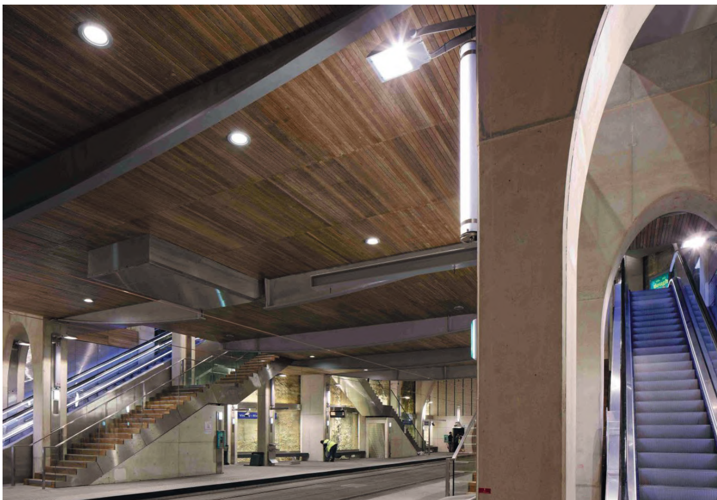
Metro Station Viroflay, Paris, France. Luminaire: 153 ©Hugo Hébrard
